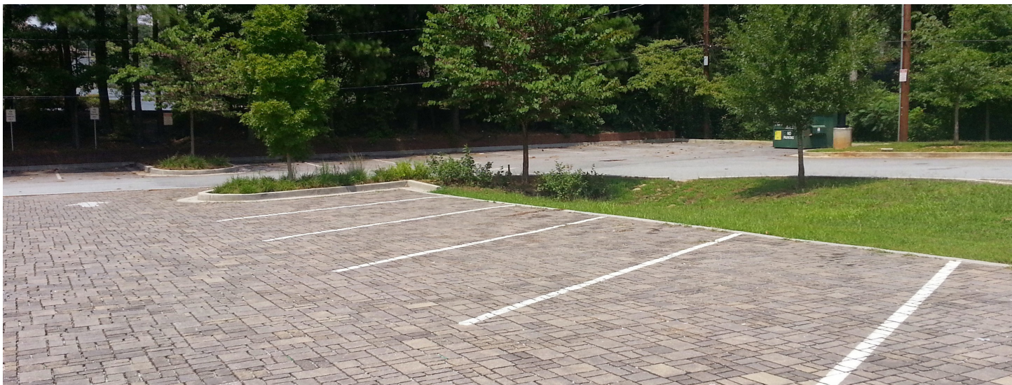
An example of pervious pavement used as a best management practice (BMP) to mitigate stormwater runoff at the Toco Hill-Avis G. Williams Library, Dekalb County.
