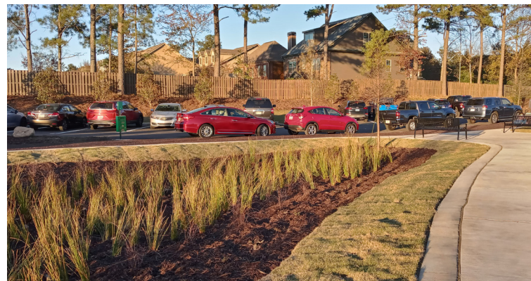
Example of a rain garden adjacent to parking used to treat stormwater in Johns Creek, GA.
