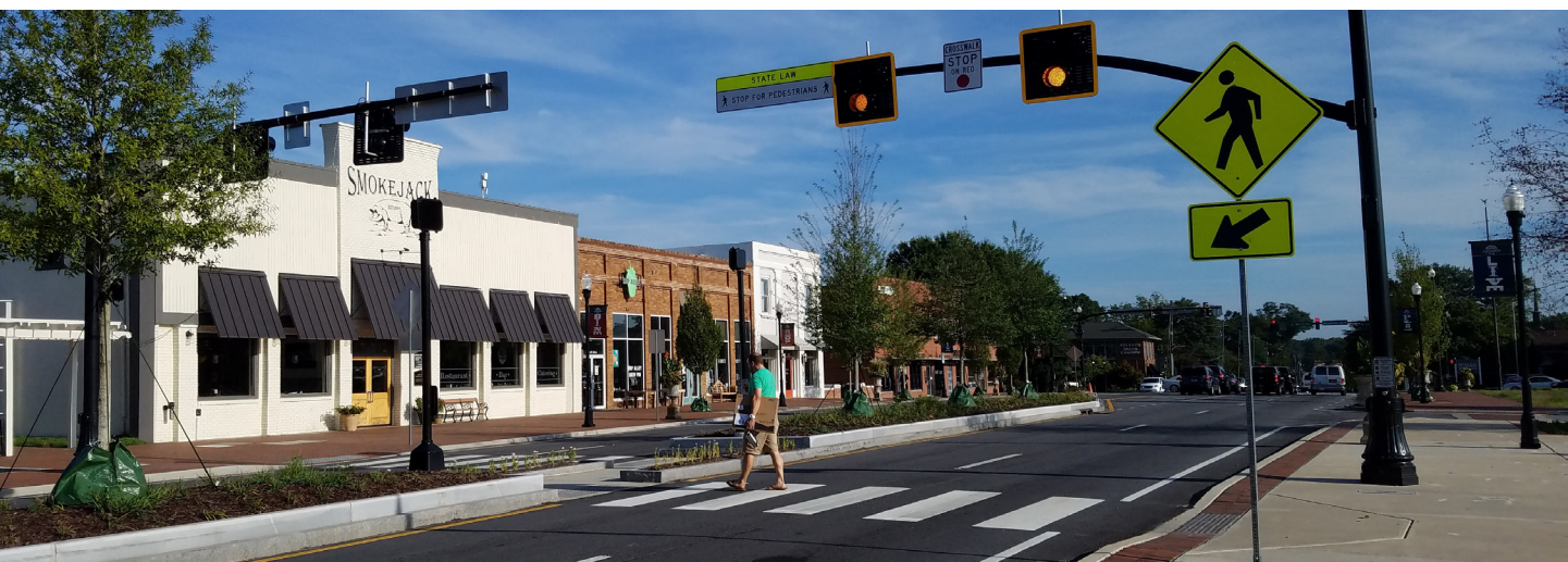
The Garden Walk Alignment proposes a mid-block crossing. It is recommended that the crosswalk be designed with a HAWK signal and a refuge island, like the one pictured above located in downtown Alpharetta.
