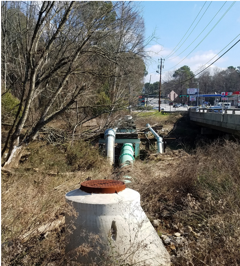
Large utility pipes crossing the Flint River at this potential terminus for the model mile could pose complications during construction.
