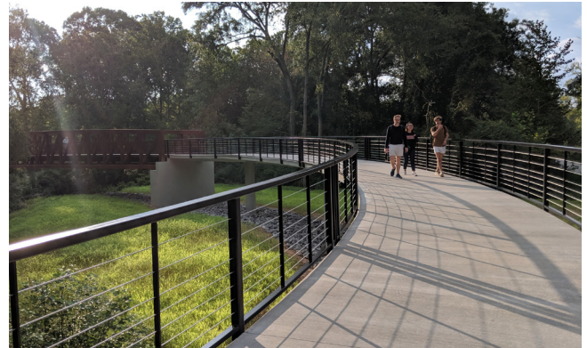
An example of a boardwalk with concrete decking and a decorative metal safety railing.
