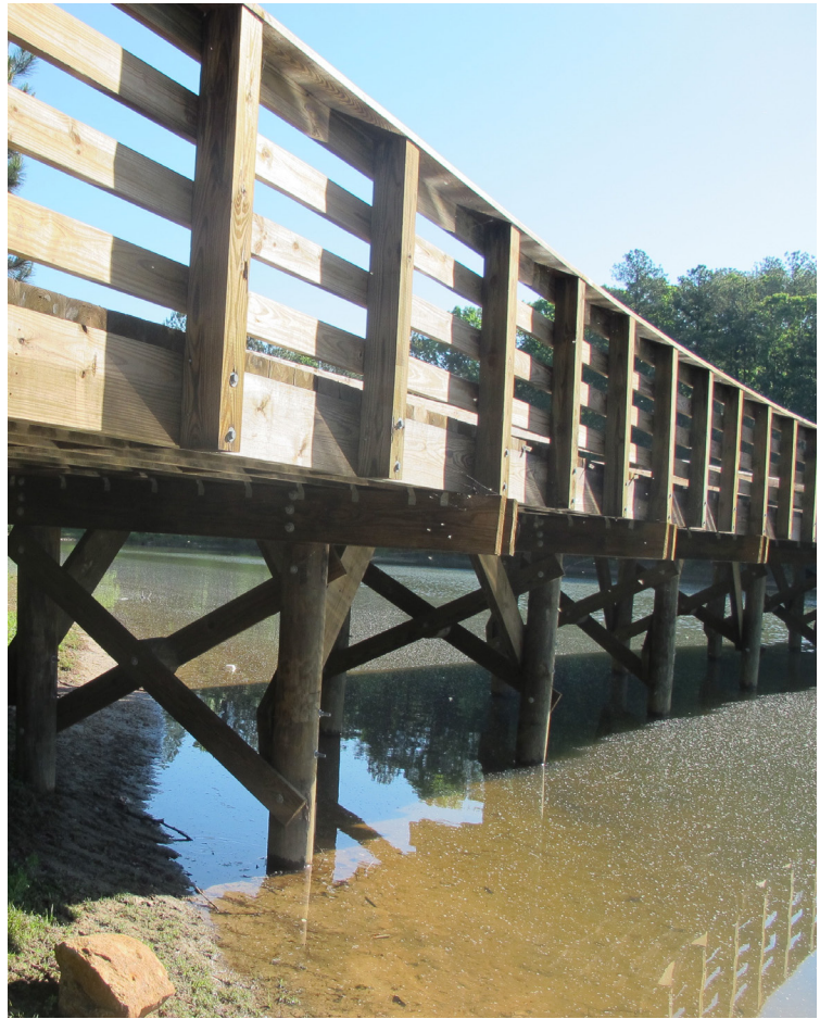
A segment of the Wetland Walk Alternative proposes a raised boardwalk through wetlands, similar the International Park boardwalk pictured above. It is recommended that top-down construction methods be used to protect the wetlands.
