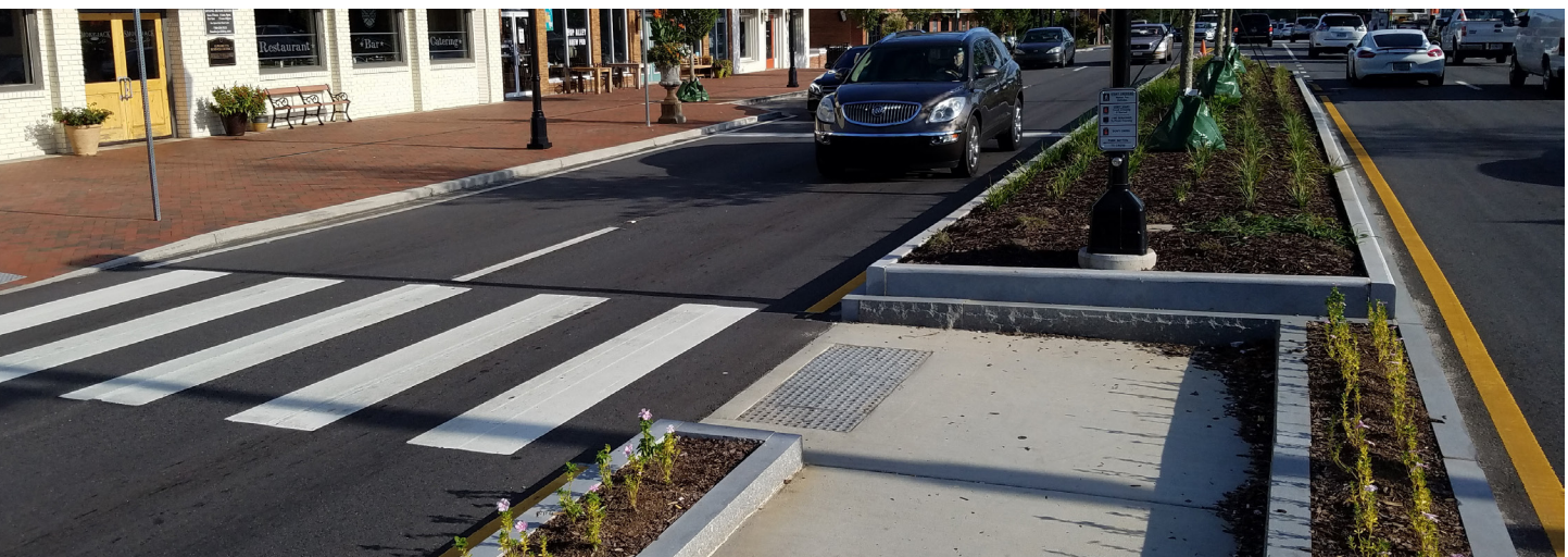
The School Walk Alignment proposes a mid-block crossing. It is recommended that the crosswalk be designed with a HAWK signal and a refuge island, like the one pictured above located in downtown Alpharetta.
